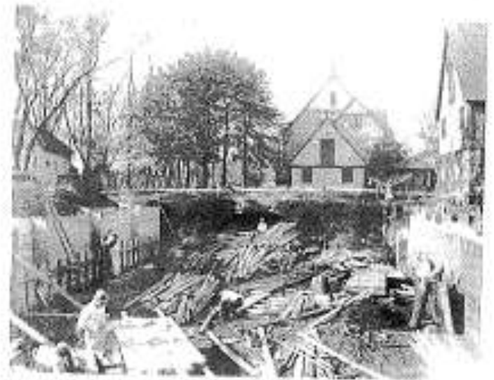
Building the new Parish House (Hanks Memorial), south side
